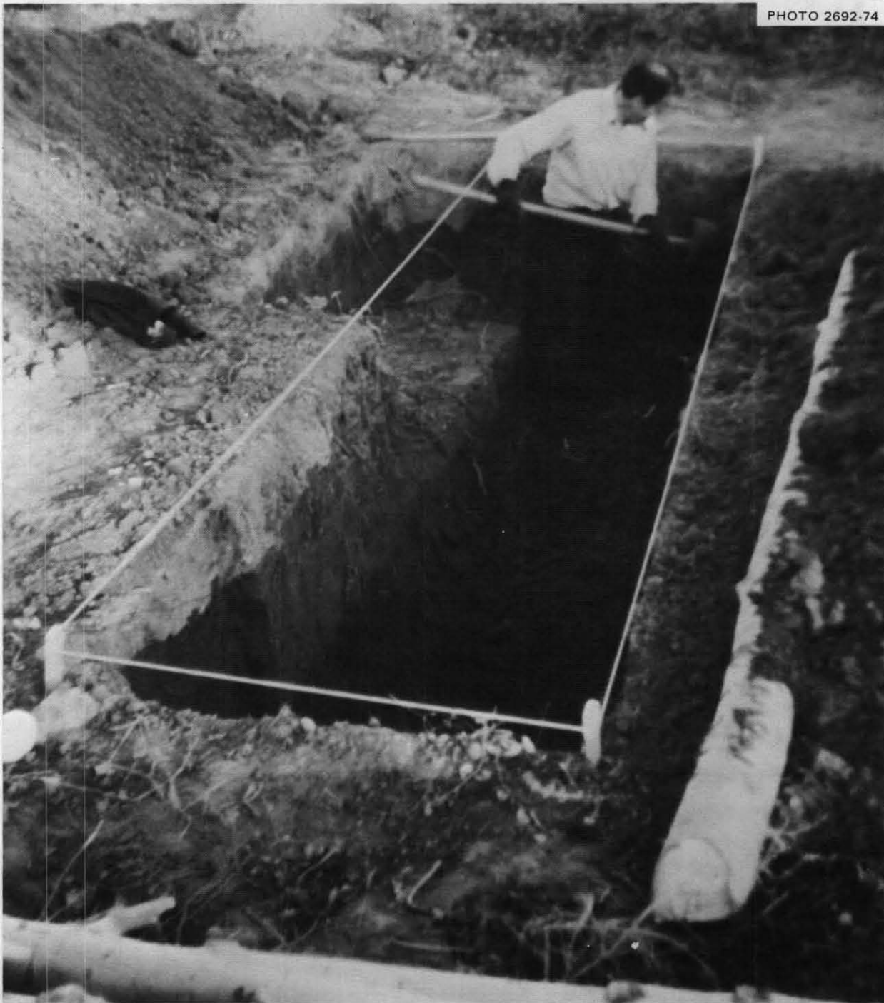
Fig. 4.4. Expanding the shelter room to its full specified width of 3\frac{1}{2} feet, and to its 4\frac{1}{2} -ft depth. This intelligent man made unnecessary work for himself by not following the instructions to cut a 3\frac{1}{2} -ft stick, and then use it repeatedly to be sure the trench was being dug full width.
